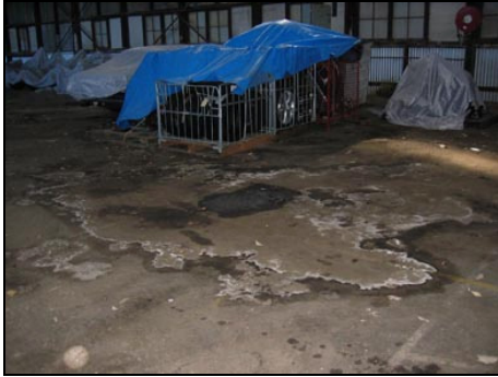
Photograph 35 – Warehouse 2 (interior) holes in roof lead to flooding of facility and possible damage to evidence
