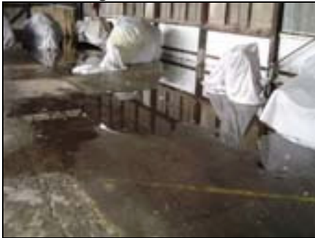
Photograph 35 – Warehouse 2 (interior) holes in roof lead to flooding of facility and possible damage to evidence
